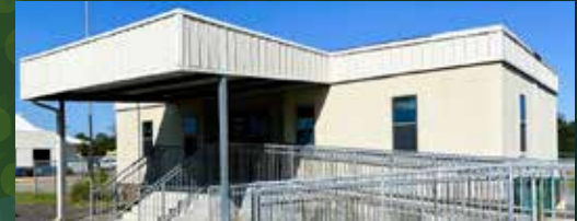
24' x 44' modular building previously used as a substation for the Calcasieu Parish Sheriff Department. It is being sold to be moved. This is a 2-piece modular building and is located at 4525 Highway 27 south of Sulphur. The concrete steps and awning areas are not included. This building has had some storm/water damage. Contact Mike Johnson at 337-263-3813 to schedule a pre-sale inspection.
